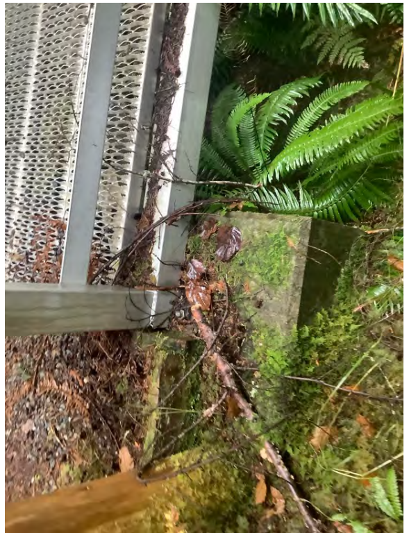
Right Bank Abutment when facing downstream
