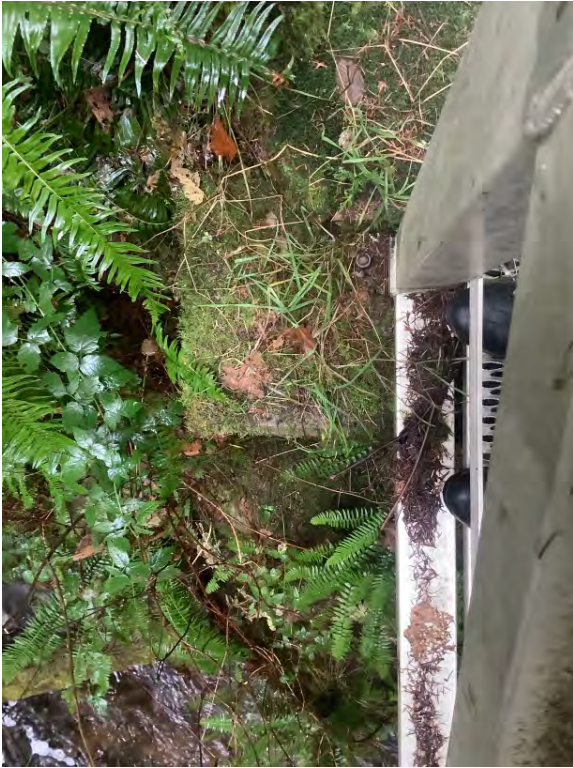
Left Bank Abutment when facing downstream
